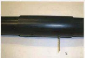
the joint sleeve and joint pipe and tighten using the supplied screw.
